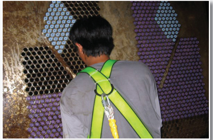
Worker loads Conco Tube Cleaners into tubeshield at Masinloc Power Station.
